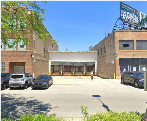
Site: View from Front
